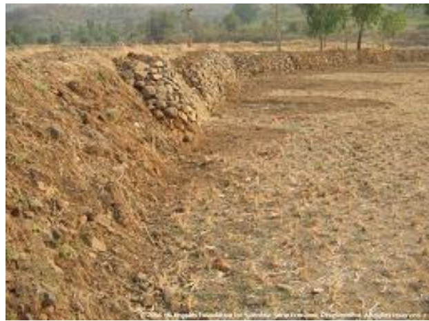
Figure 12: Damaged boundary has been fixed (Dehrang)
