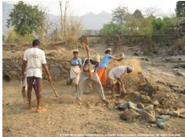
Figure 10: Work in progress at Dehrang
